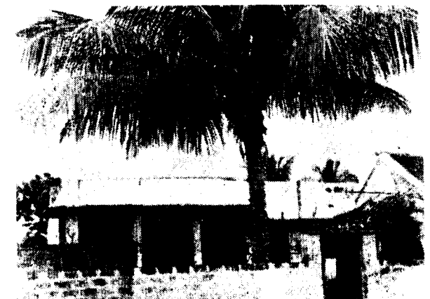
Building Donated by No. 2 to Peetadhipati at Durgapuram, Vijayawada
