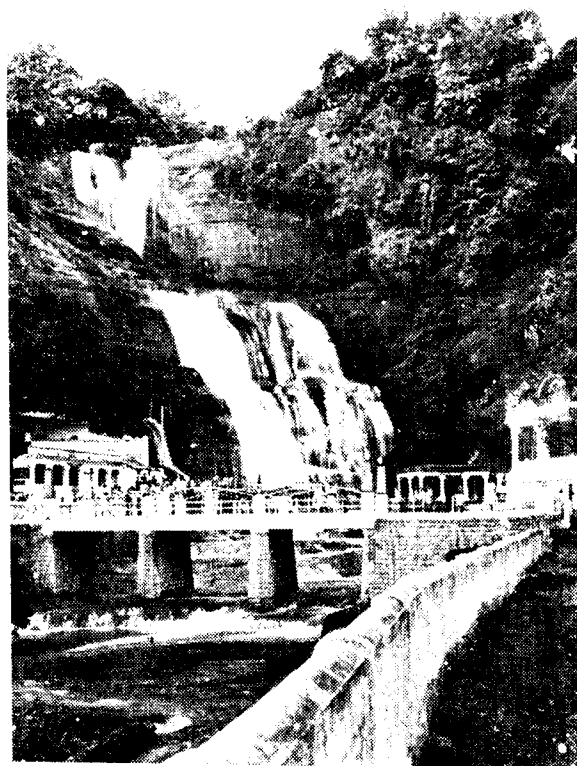
Main water falls in Courtallam
