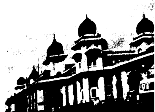
Egmore Railway Station.
