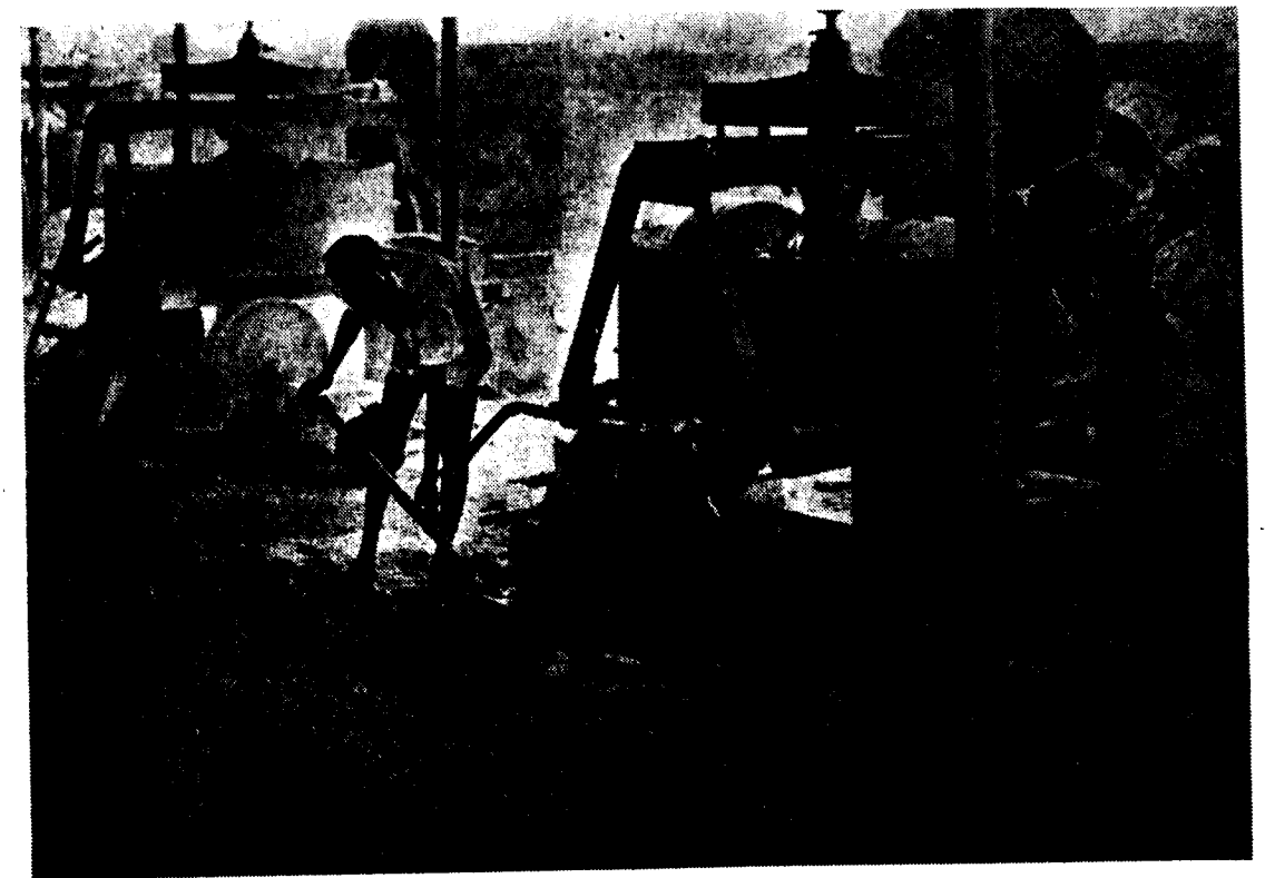
Mortar Pan mixer, working at the Board's Lime Yard at Kodambakkam Pudoor.
