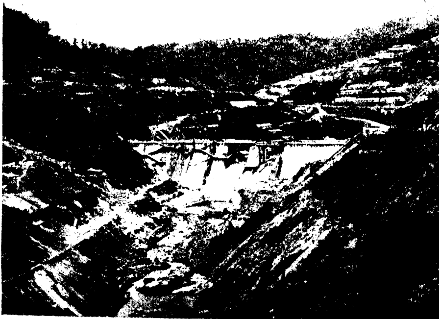
KUNDAH HYDRO-ELECTRIC SCHEME Kundah Forebay Dam.
