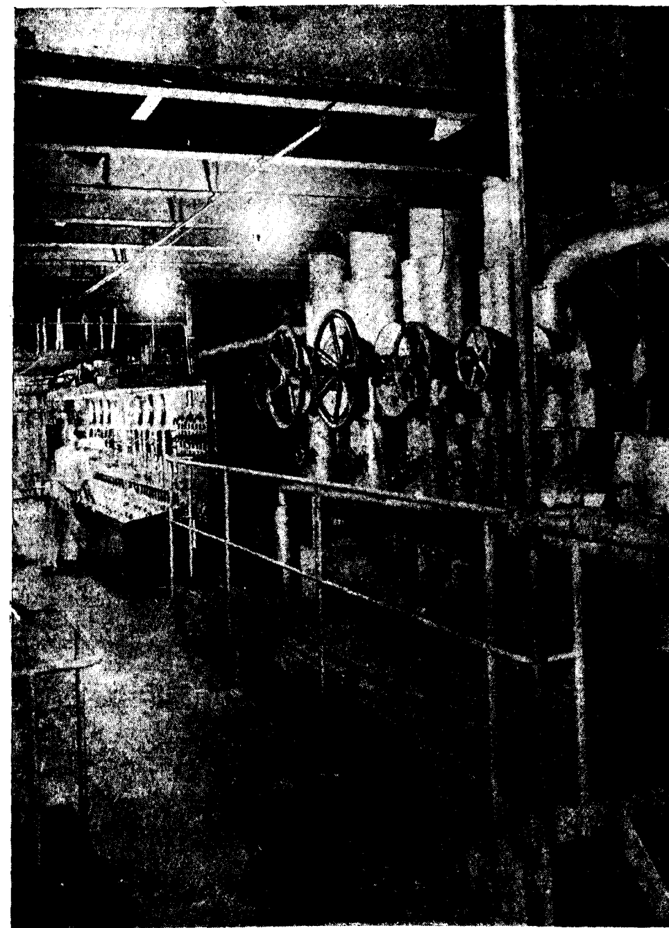
BASIN BRIDGE POWER STATION. View of Askania control with main steam distributor and valves.
