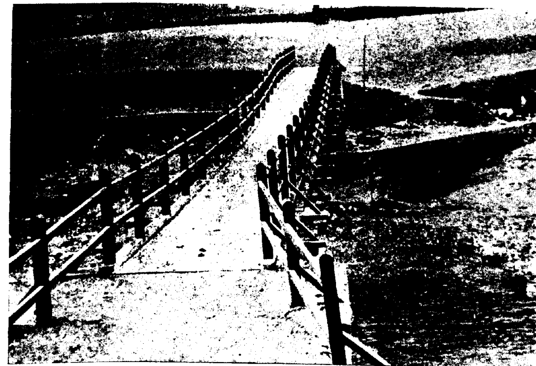
The Bhilo Bridge over a rivulet in Chamba District built under the Tribal Welfare Scheme—Himachal Pradesh.
