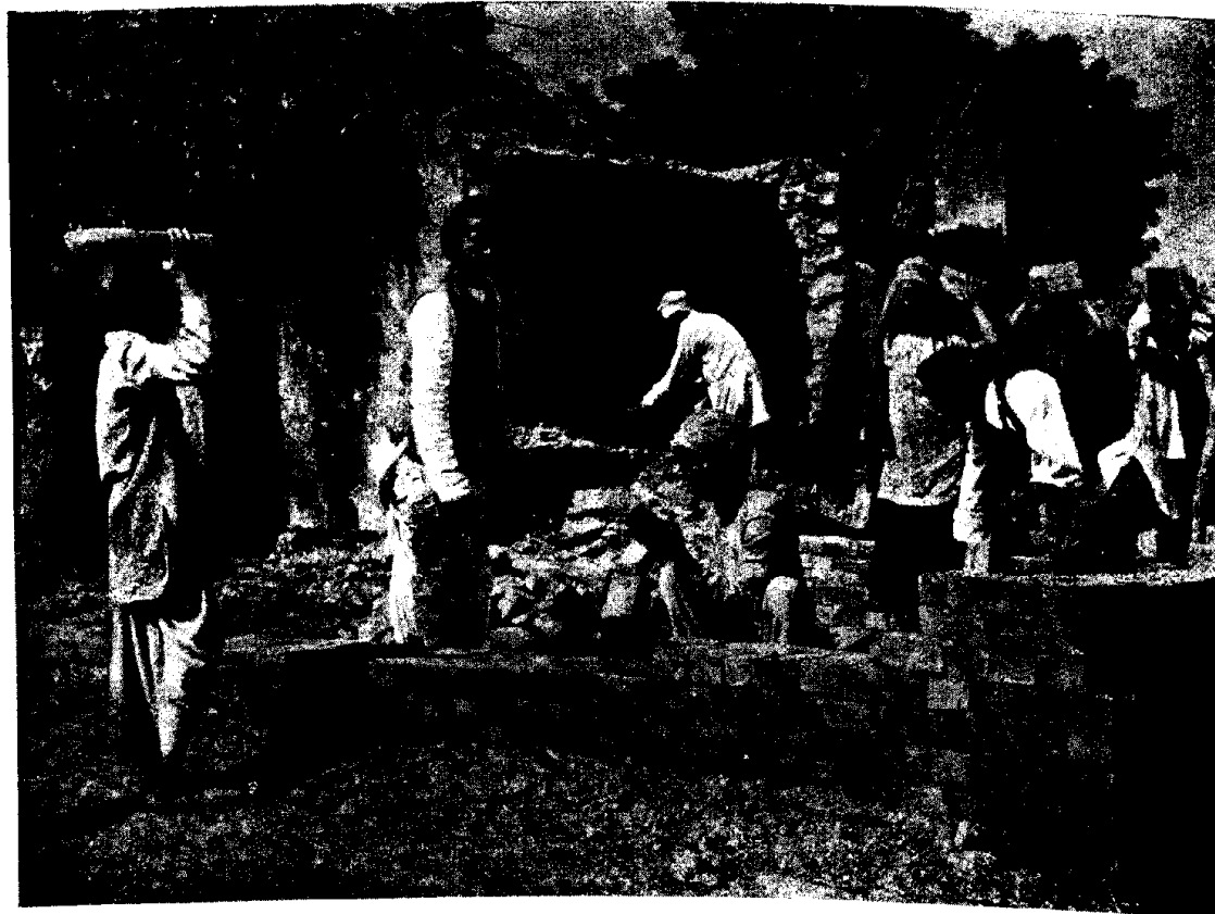
New Houses for old—harijans building their own houses under the subsidised housing scheme—Delhi.
