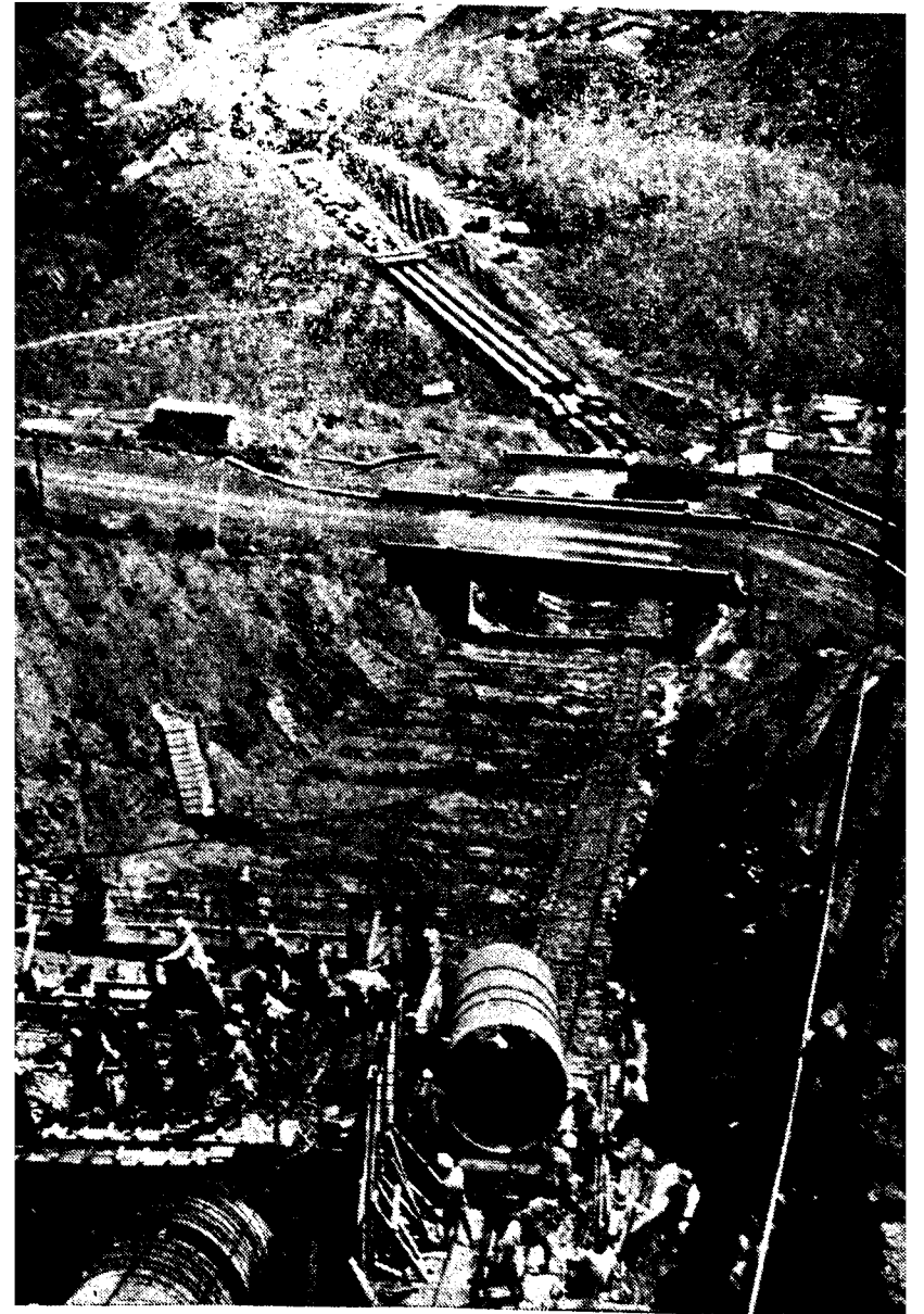
PERIYAR PENSTOCK BRIDGE FACING DOWN WITH PENSTOCK PIPES.
