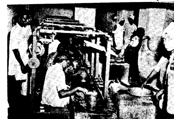
SILK REELING INDUSTRY. IMPROVED METHOD OF SILK REELING.
