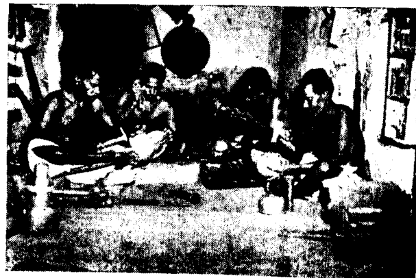
SHAPING LEAD WARES.
