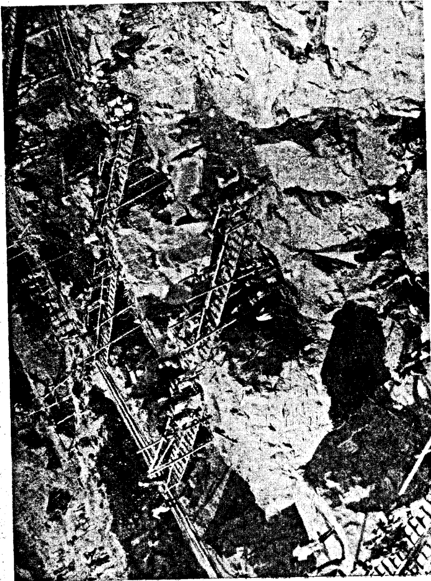
PERIYAR—POWER HOUSE EXCAVATION FROM NORTHERN CORNER OF P.H.
