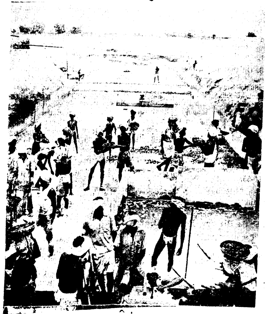
FIG. III (G).—CONSTRUCTING A CAUSEWAY ACROSS PENNAR NEAR MELAPATTAMBAKKAM FINISHING CONCRETE IN DEEP VENTED PORTION.
