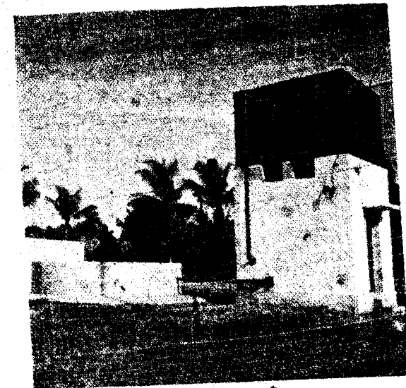
Over head tank and well (Kodambakkam Rehousing Scheme)
