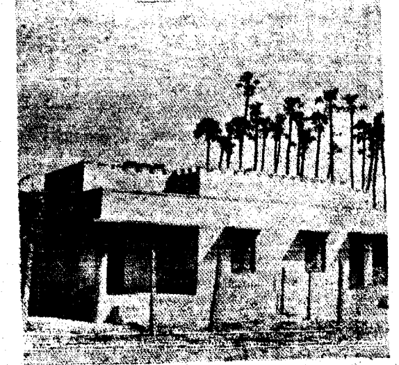
Semi detached building with brick masonry walls and T. Beam roofing, as per design No 11-A/51 (Mambalam South Area Scheme), Plinth area 1315 sq. ft.—Cost Rs. 8600.
