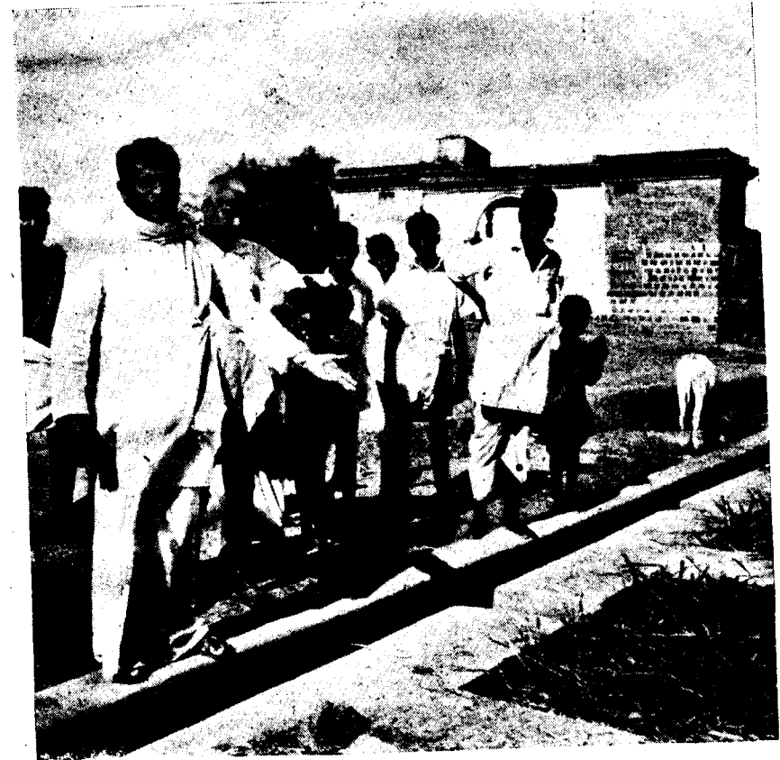
A village drainage constructed by the villagers themselves with technical assistance given by the Government—The Rural Welfare Officer will be seen explaining how waste can be converted into wealth.
