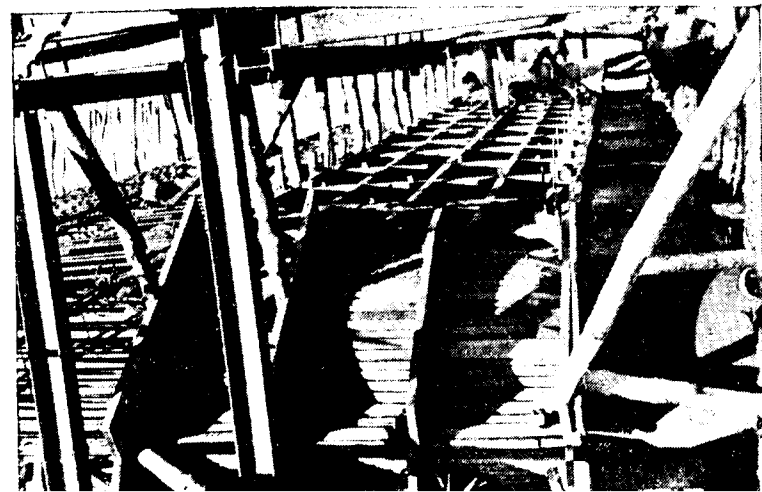
FIG. III (E).—NOYYAL BRIDGE. FIGURE SHOWS THE FRAMEWORK FOR THE L.E. 8 WITH R.S. JOISTS WHICH SERVED AS SCAFFOLDINGS.
