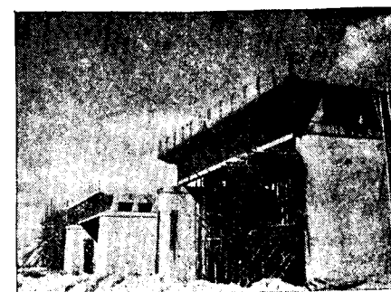
FIG. III (M). CONSTRUCTING A BRIDGE ACROSS THE RIVER PENNAE NEAR NELLORE ON MADRAS-CALCUTTA ROAD—N.H. 5.
