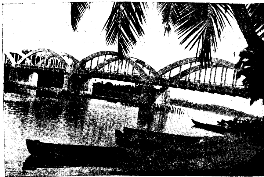
FIG. III (B).—BRIDGE OVER THE GURPUR RIVER NEAR KULUR AT M. 4/7-8 OF MANGALORE-BAINDUR ROAD.
