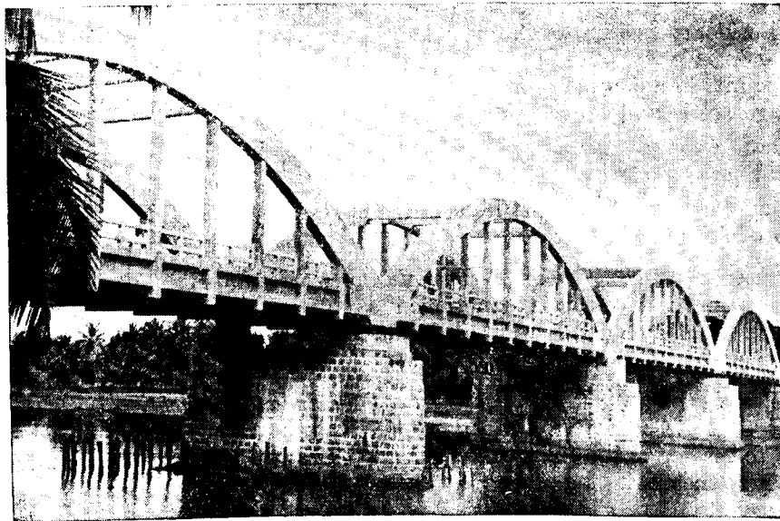
FIG. III (A).—BRIDGE OVER THE GURPUR RIVER NEAR KULUR AT M. 4/7-8 OF MANGALORE-BAINDUR ROAD.
