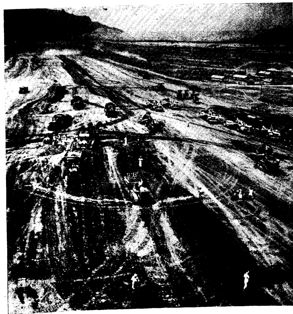
LOWER BHAVANI PROJECT JANUARY 1952—EARTH DAM IN FORMATION.
