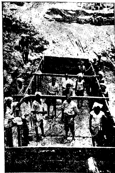
FIG. III (k).—OPEN CAISSON READY FOR SINKING INTO SANDY SOIL (PIER NO. 17).
