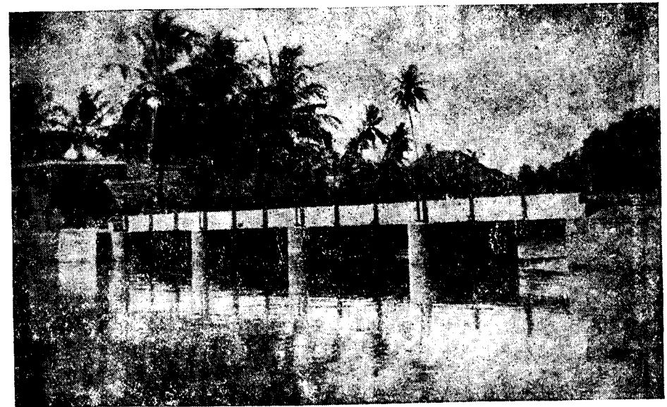
FIG. III (f).—BRIDGE ACROSS NATTAH RIVER AT MILE 10/1 OF KONERIRAJAPURAM VILLAGE ROAD, 4 SPANS OF 15 FEET.
