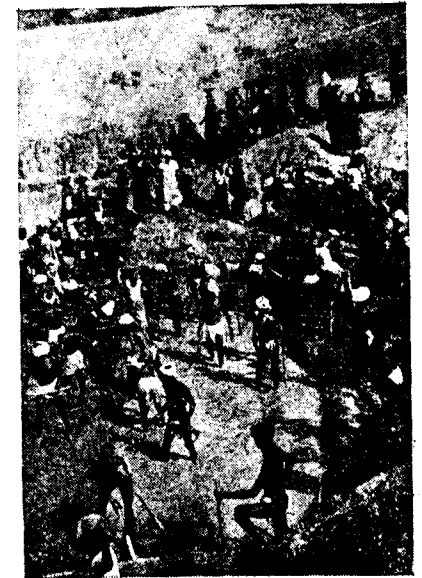
FIG. III (h).—SHOWING EXCAVATION IN VIGOROUS PROGRESS.
