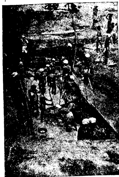
FIG. III (i).—SHOWING THE HEAVY EXCAVATION TO GET AT THE ESTIMATED DEPTH WHICH IS 15 FEET BELOW BED LEVEL (PIER NO. 9).
