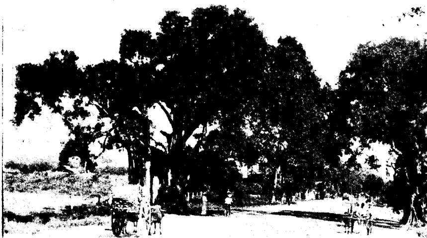
Fig. III (f).—CONPHALT WORK IN 7/5—12/0 OF G.S.T. ROAD.
