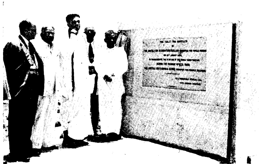
FIG. III (d).—LAYING OF FOUNDATION STONE FOR THE BRIDGE OVER THE RIVER PENNAR NEAR NELLORE ON 20TH AUGUST 1950 BY HON'BLE SRI M. BHAKTAVATSALAM, MINISTER FOR PUBLIC WORKS.
