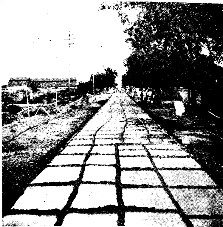
Fig. III (e).—CEMENT CONCRETING KARAUKUDI-DEVAKOTTAH ROAD, M. 52/0—57/0.
