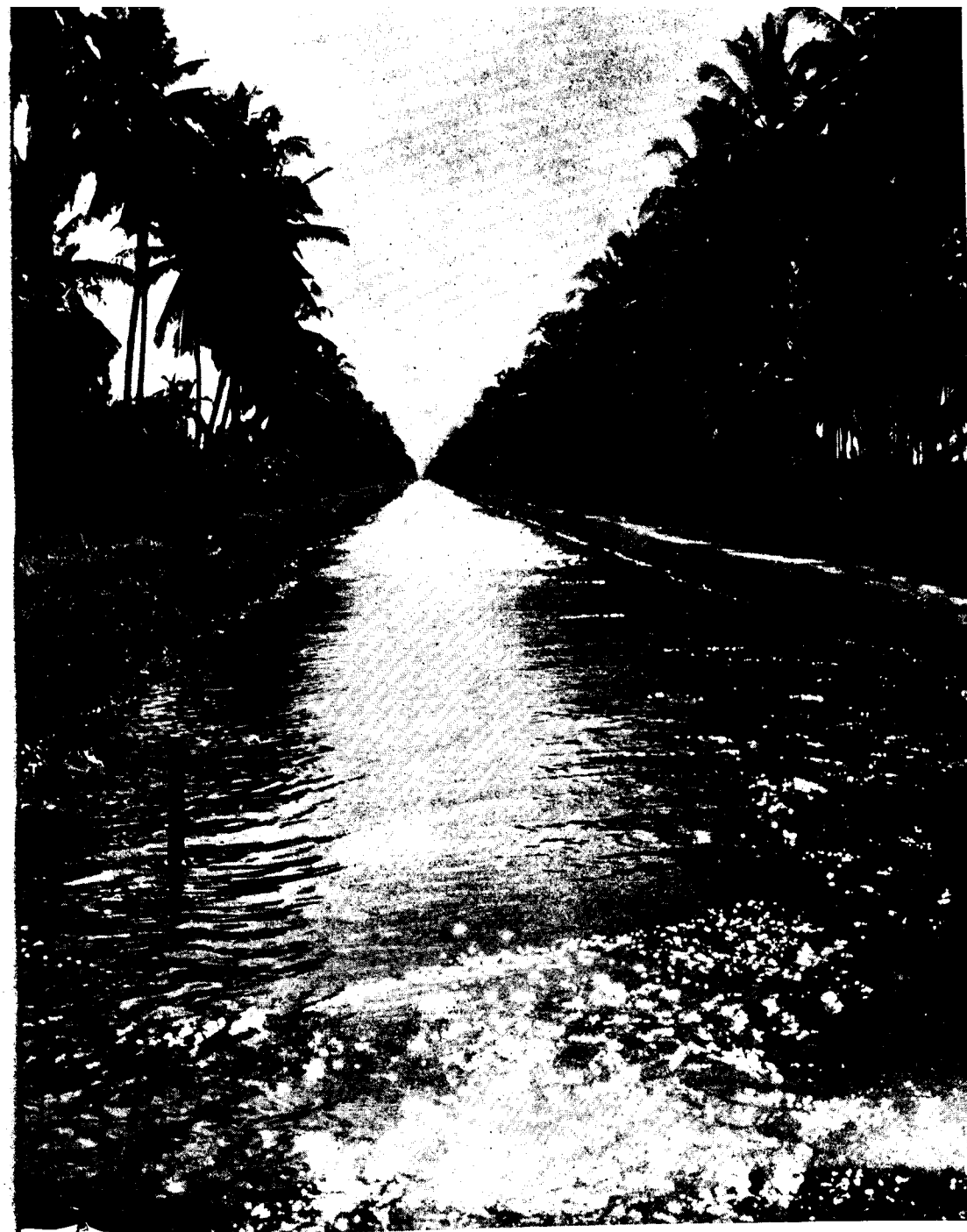
Krian Irrigation canal.
