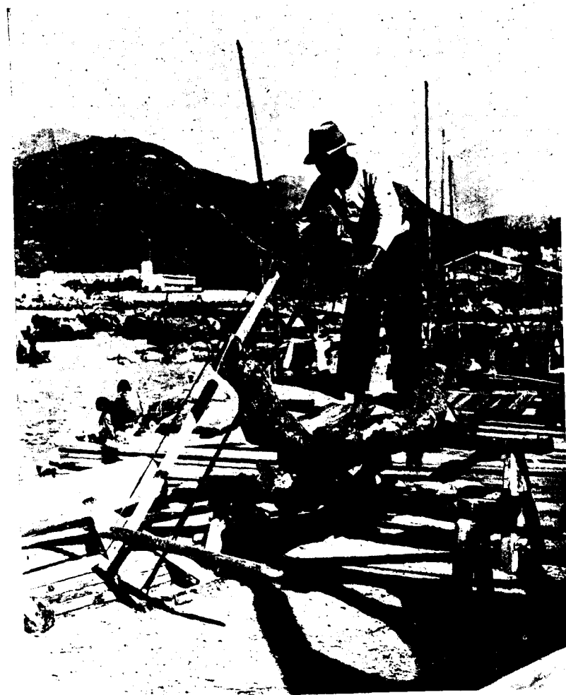
Cutting timber for junk building at Aberdeen.
