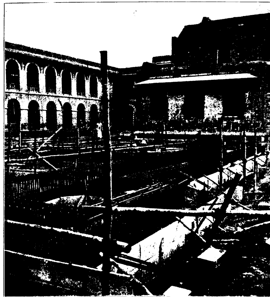
1. REINFORCEMENT FOR THE R. C. RAFT FOUNDATION TO THE PRESIDENCY COLLEGE SCIENCE BLOCK EXTENSION.
