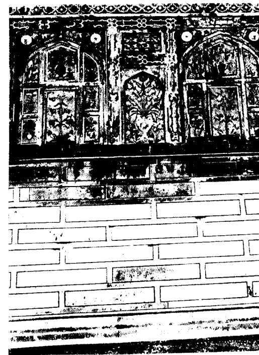
(a) Agra. The Taj. Details of north wall showing panels and ashlar masonry.
