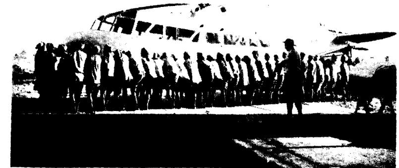
The fuselage being prepared for assembly on to its floats.
