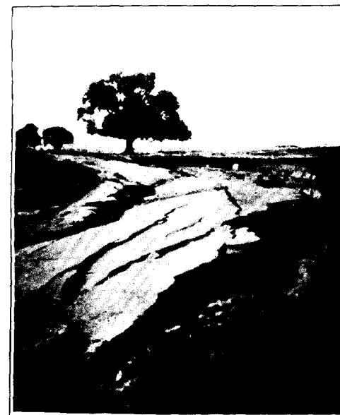
Damage to roads and bridges
