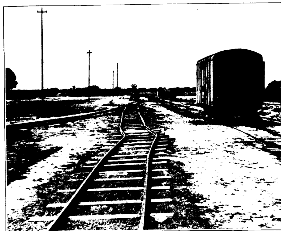
Railway track distorted laterally.
