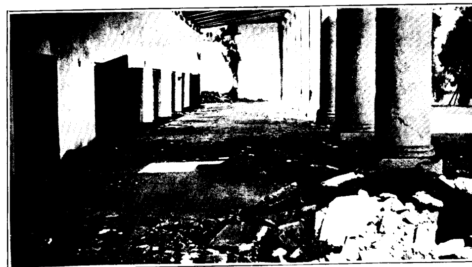
The central part of this house sank through the floor half way to the lintels of the doors.
