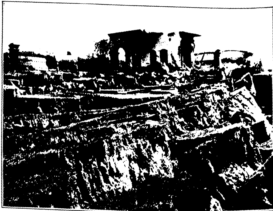
Fissures on the bank of the lake at Motihari. This was formerly level ground.
