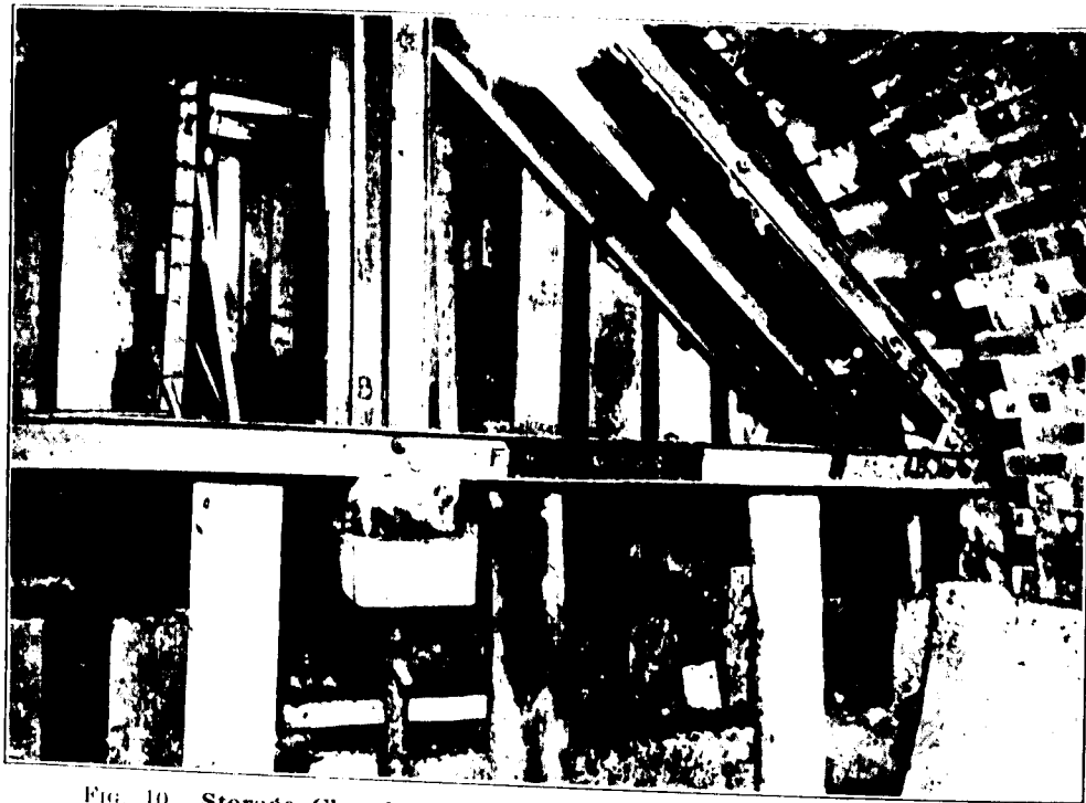
FIG. 10. Storage Chamber showing Method of Supporting Timbering.
