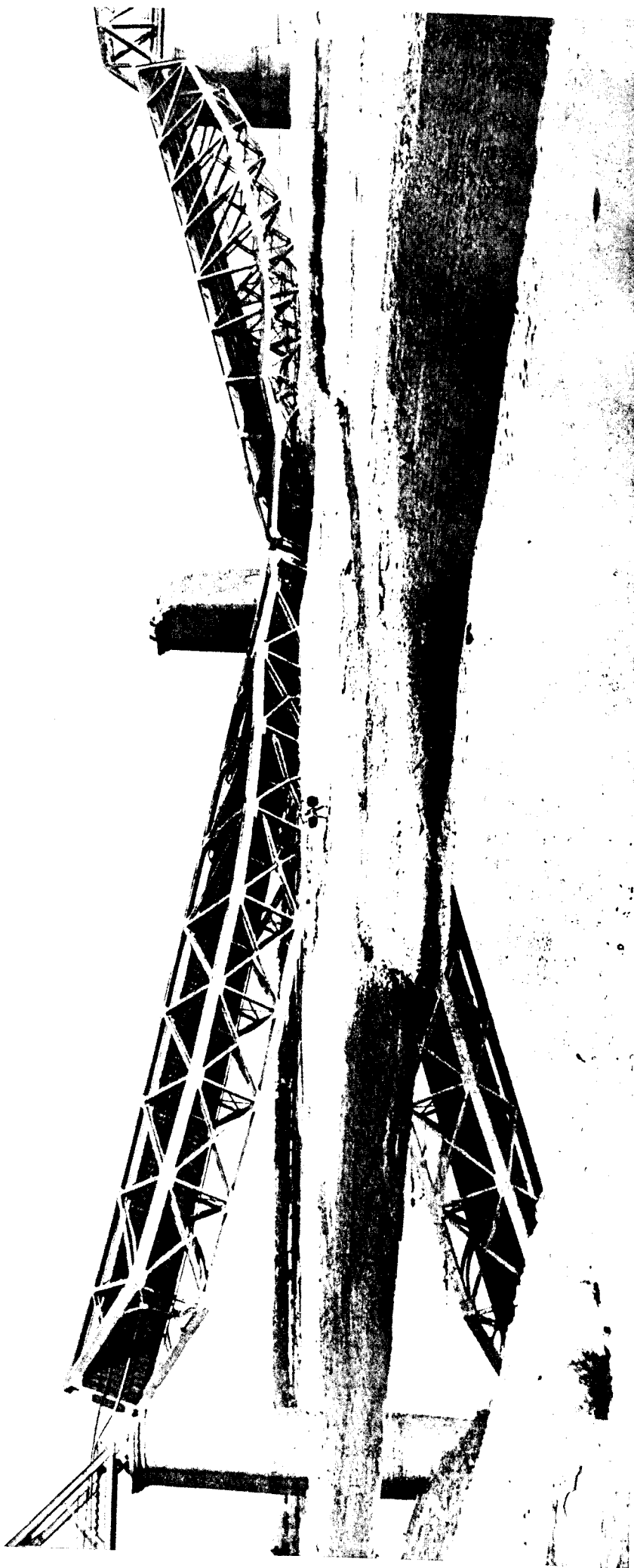
Inchcape Bridge over Gogra River, Spans Nos. 15 & 16 shaken off piers, by earthquake.
