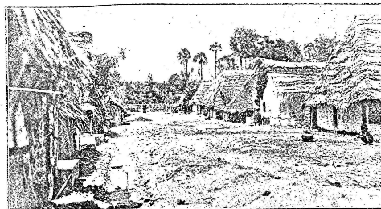
VINAYAKAPURAM HUTTING GROUND. IMPROVEMENT IN PROGRESS.
