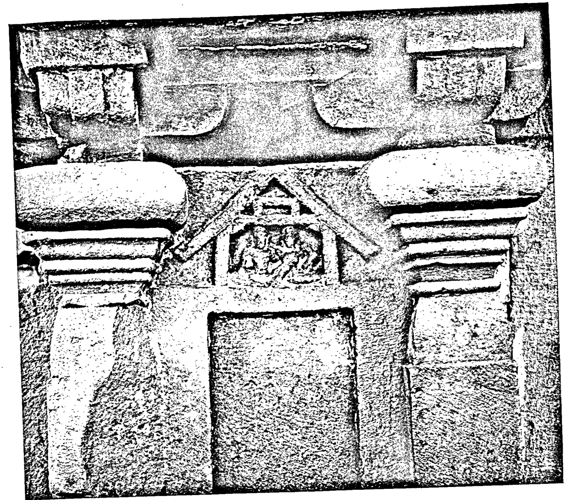
(a) BADAMI, DISTRICT BIJAPUR. SURALI OR SUVALI TEMPLE. MODEL OF A PSEUDO-QUEEN-POST TRUSS IN RELIEF ON WALL.
