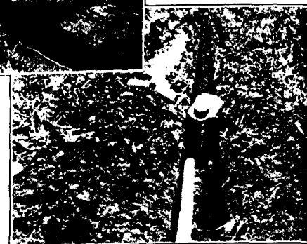
Tile drainage reduces the number of surface ditches required and is also proving a most promising solution of the problem of mosquito breeding in seepage areas and wet lands in Porto Rico.
