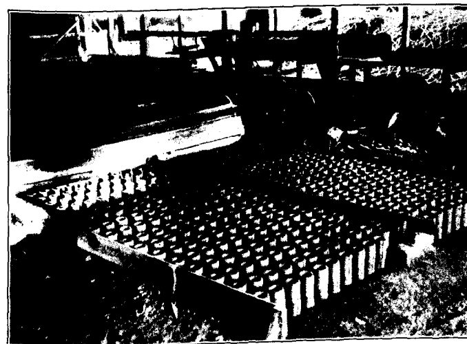
Tiles manufactured in Porto Rico for the subsoil drains which are being installed in connection with antimalaria work. Local manufacture of the tiles greatly reduces the cost of the drainage projects.
