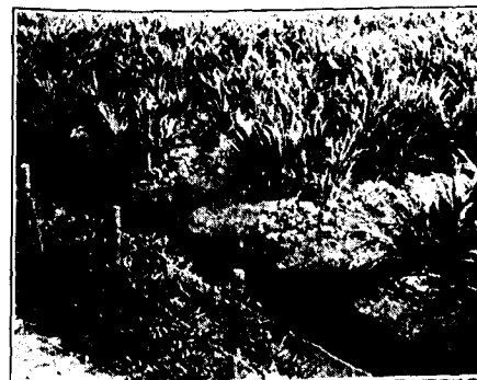
Tile drainage reduces the number of surface ditches required and is also proving a most promising solution of the problem of mosquito breeding in seepage areas and wet lands in Porto Rico.
