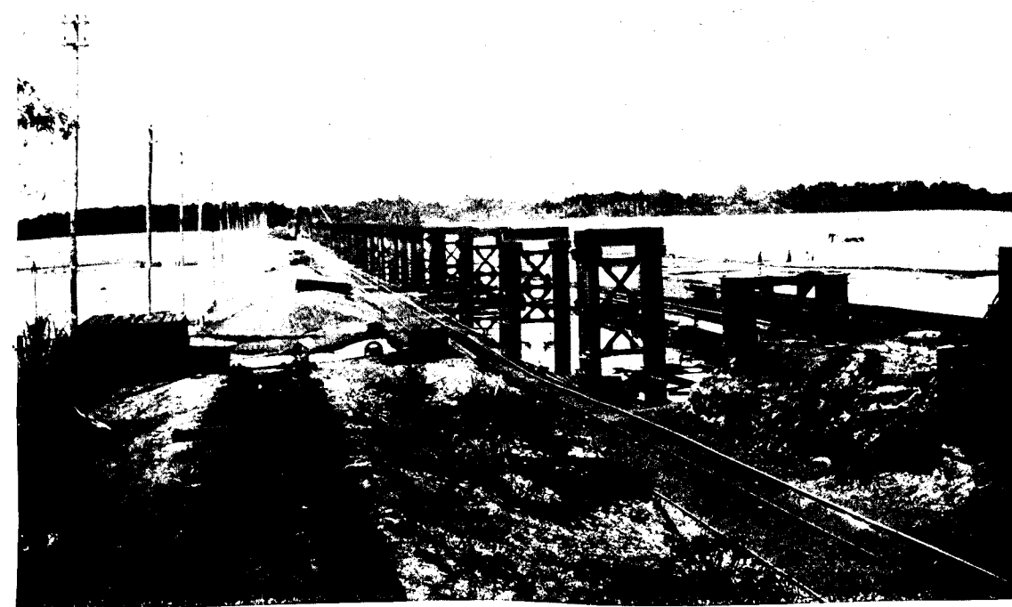
SHOWING OPERATIONS AT THE 39TH SPAN.
