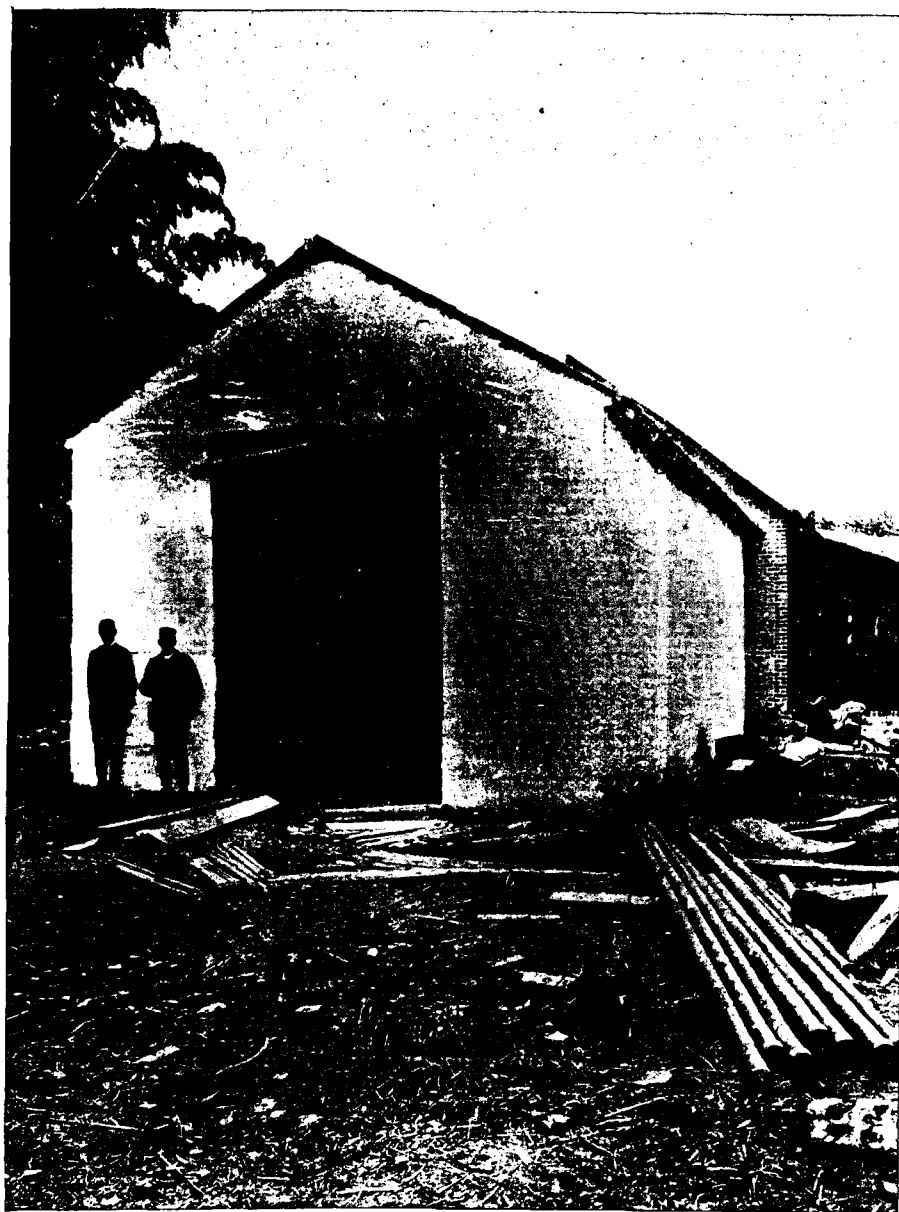
Photo I. A kiln similar to the above has a capacity of approximately 8 tons of box shooks or 2 tons output per day, and may be built for Rs. 5,000 exclusive of the power plant. Its greatest usefulness is probably in connection with small semi-portable saw mills operating in the jungle.
