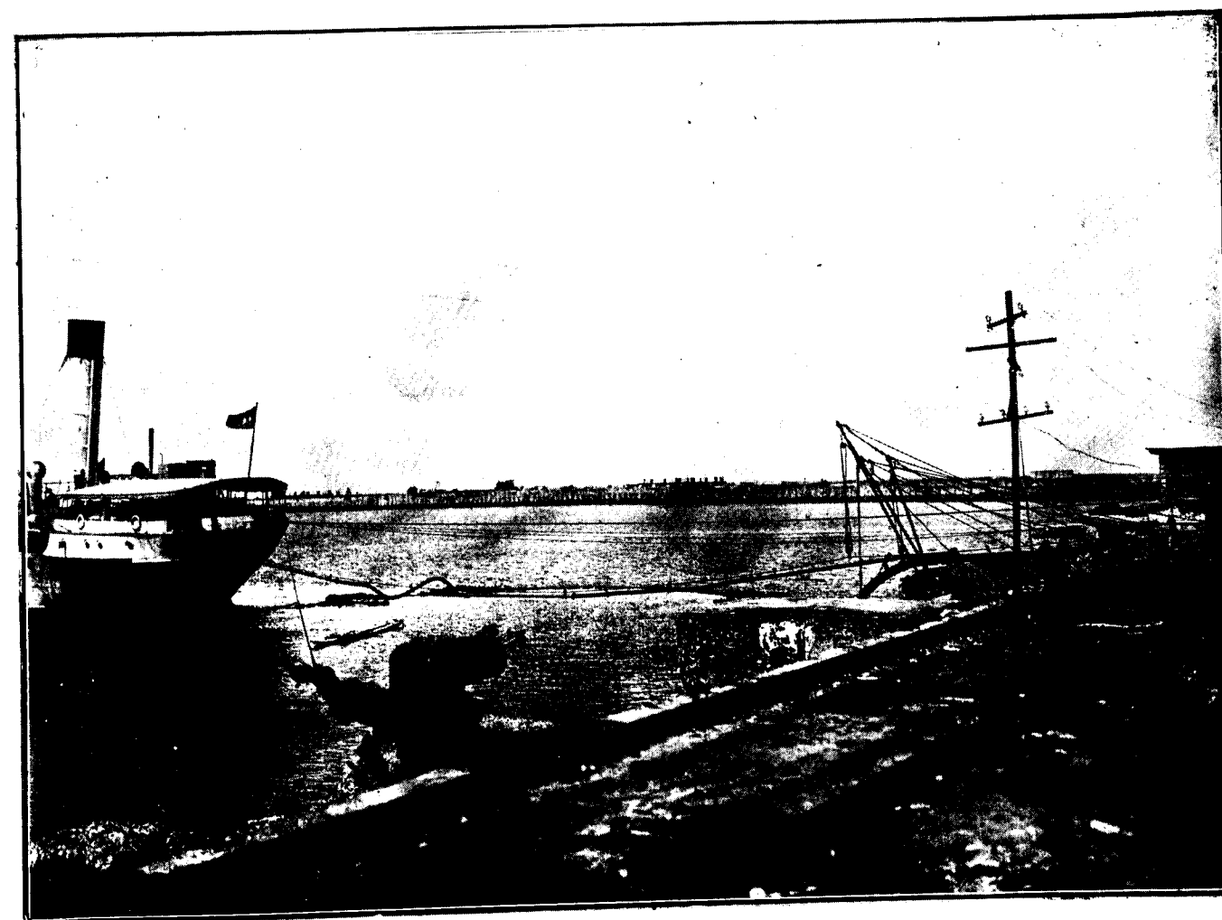
VIEW OF SUSPENDED STEAM PIPE AND FLOATING OIL PIPE.
