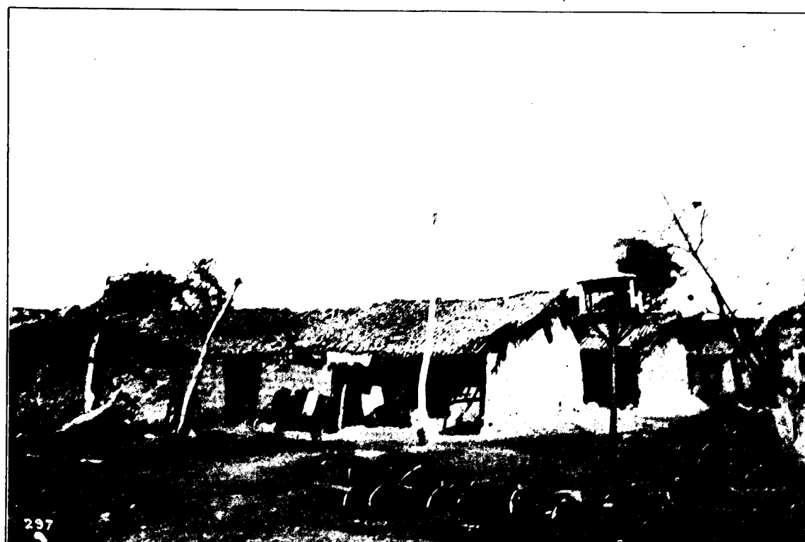
Ahmedabad—Hut built of brick and mud masonry. Occupied by Mill hands. In one of the rooms (11' x 11' x 10') there were 8 inmates residing.
