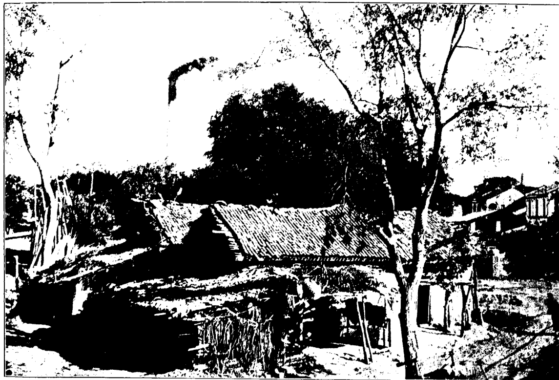
Some huts occupied by Mill hands in Ahmedabad. Rent of the very kutcha shed in front is Re. 1 per month. Built of bamboo battens mostly unplastered. No privy or water convenience.
