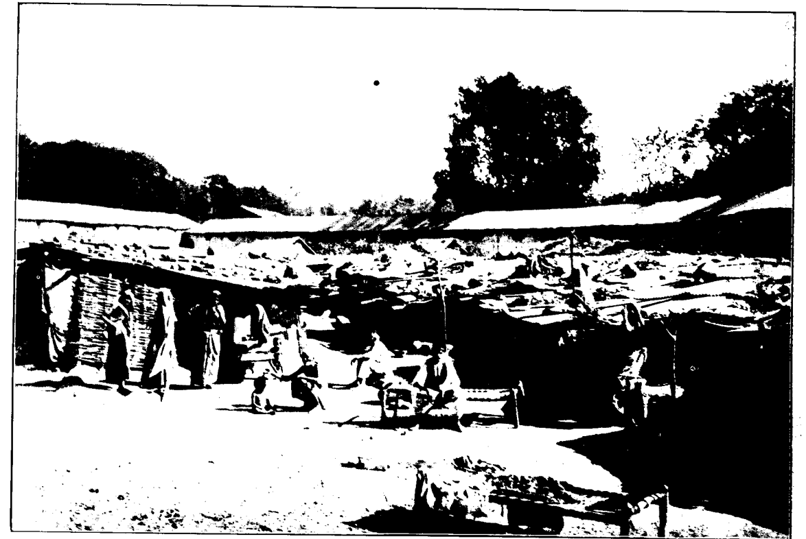
Very primitive tin sheds used for Housing of Mill Employees in Ahmedabad. Note the rubbish on roof. Size of room 10' x 8' 6". Height only 6' 0". Four to six persons stay in each so called room. Rent annas eight per month.
