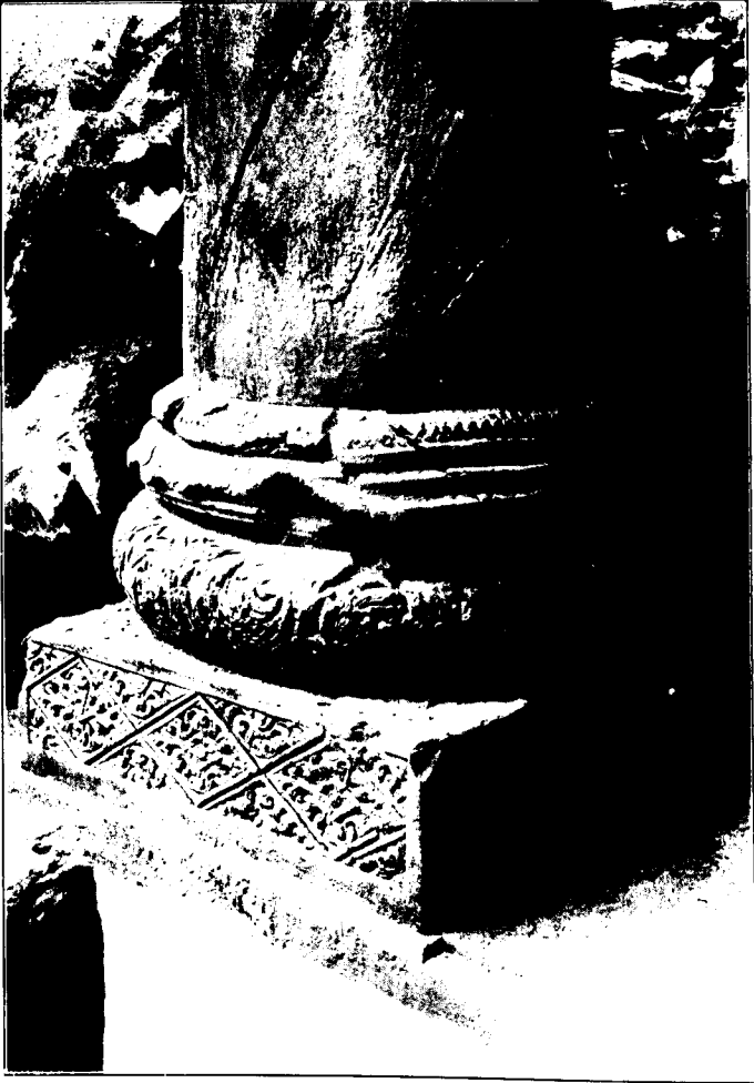
d. BASE OF MANDAPA PILLAR.
