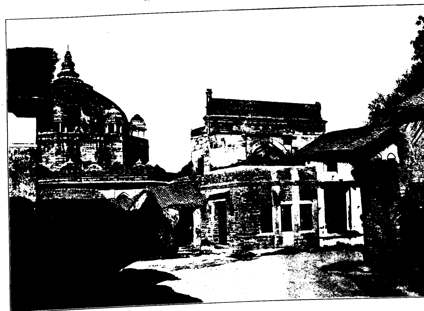
a. BEFORE REMOVAL OF MODERN HOUSES.
