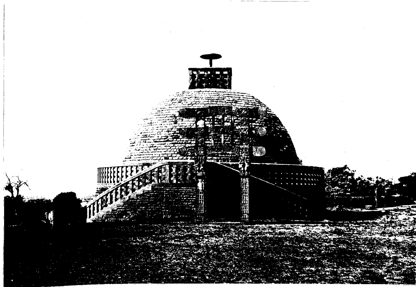
a. STUPA 3: GENERAL VIEW FROM SOUTH.
