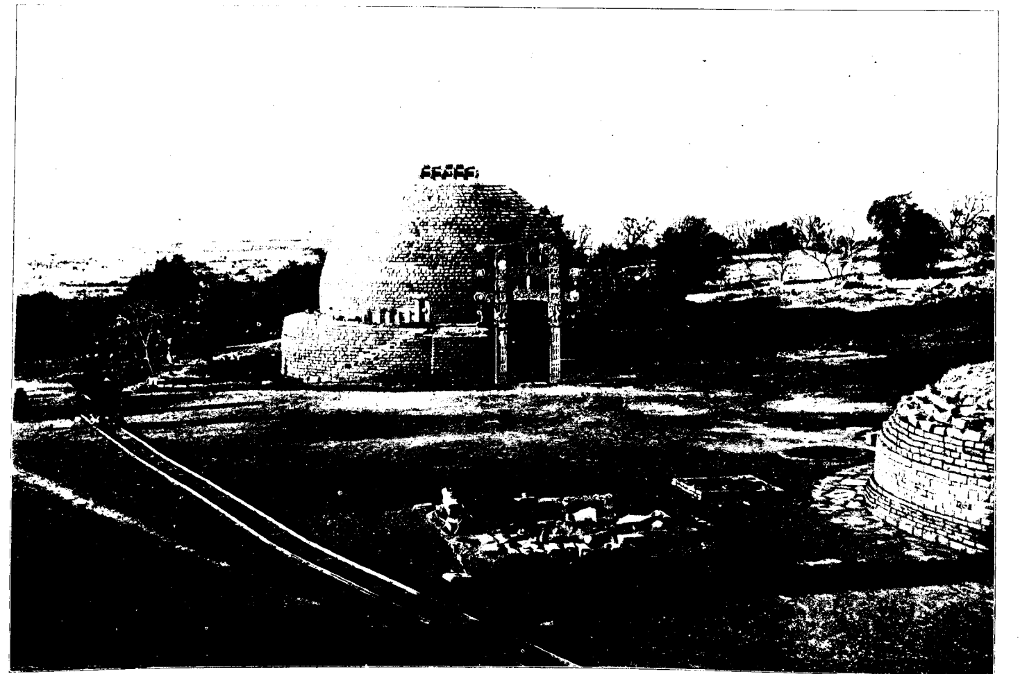
b. STUPA 3: IN COURSE OF REPAIR.
