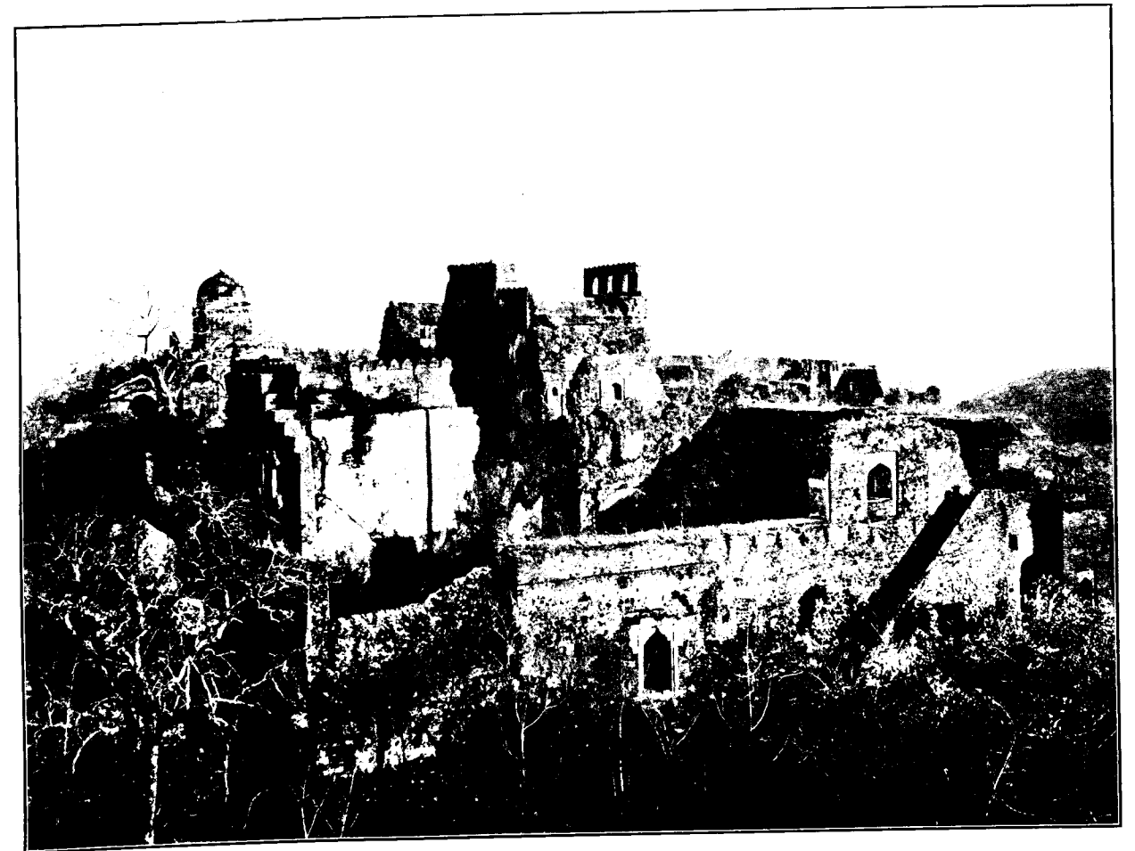
(a) CHHINDWARA: GENERAL VIEW OF DEOGARH FORT.
