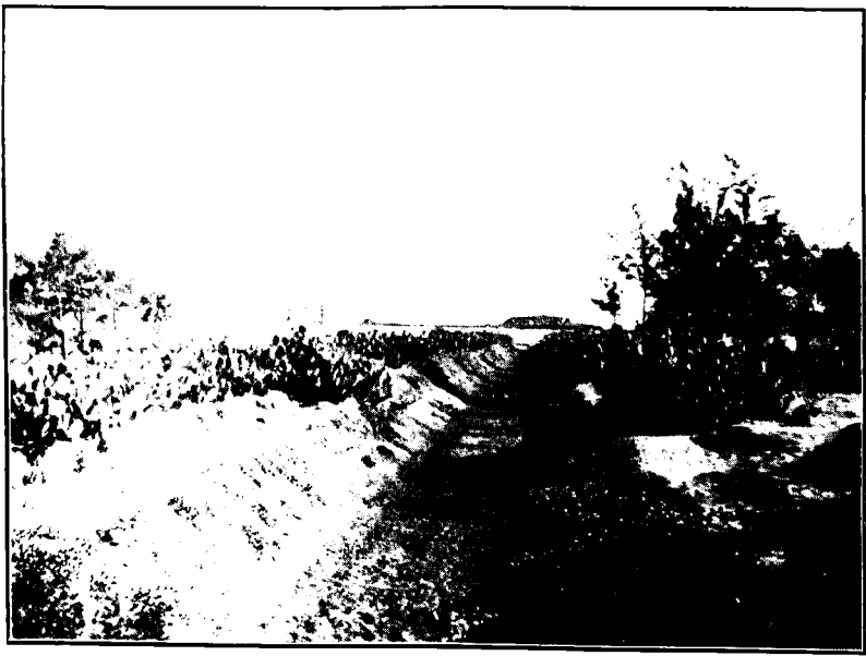
Same but at outfall: here drain is very much silted: no sullage reaches this distance except after rain fall,
