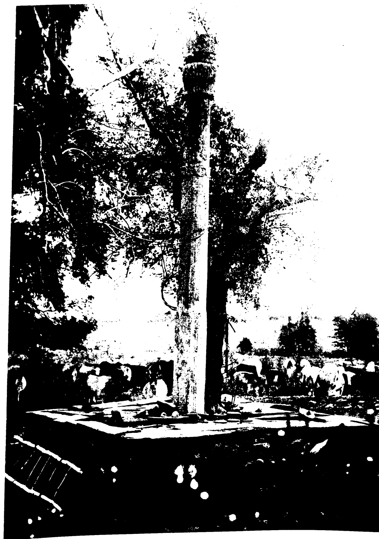
THE GARUDA PILLAR OF BESNAGAR.
