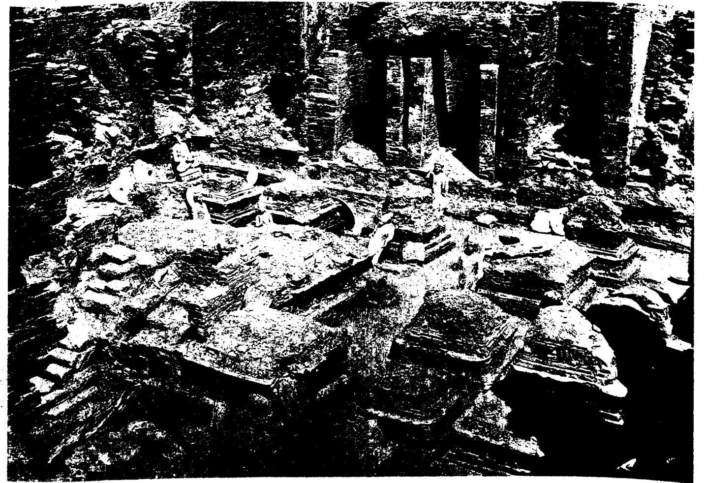
b. COURTYARD B. AFTER EXCAVATIONS (LOOKING N.E.)
