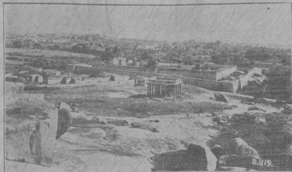
Fig. 103.—The Buildings in HAMPI.
