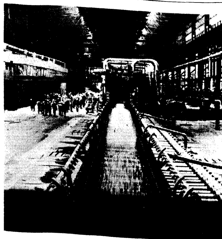
Hot strip mill of Bokaro Iron and Steel Plant built with Soviet assistance
