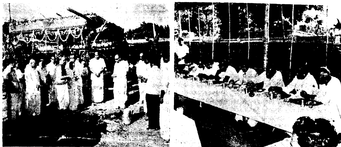
Foundation for Head office building
