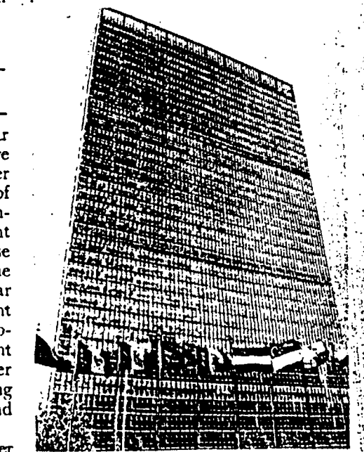
The ceiling is still too high
