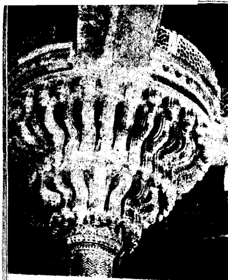
Capital of Central Column
