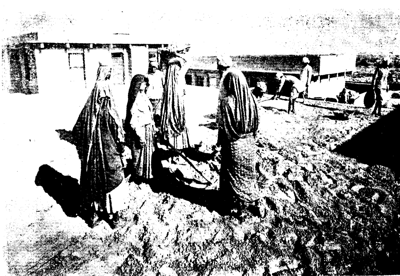
Workers engaged in the levelling of ground
