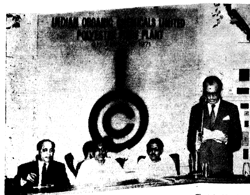
Mr. M. Karunanidhi laid the foundation for a Polyester Fibre Plant in Manali near Madras. Picture shows Mr. B. M. Ghia, Chairman of IOCL, delivering the welcome speech. Others (L to R): Messrs. D. S. Dalal, S. Madhavan and M. Karunanidhi
