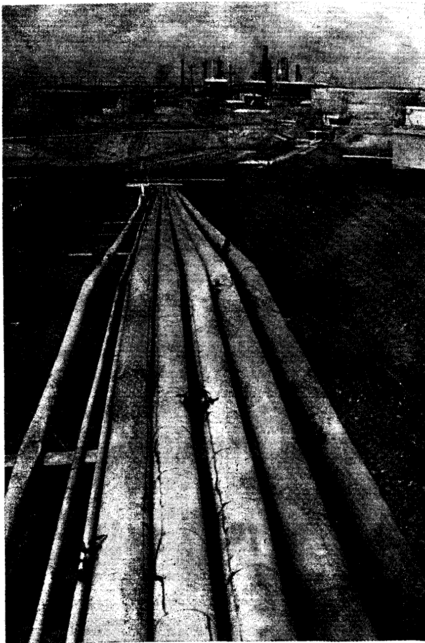
Pipelines leading to the Refinery, In the background can be seen the main plant.
