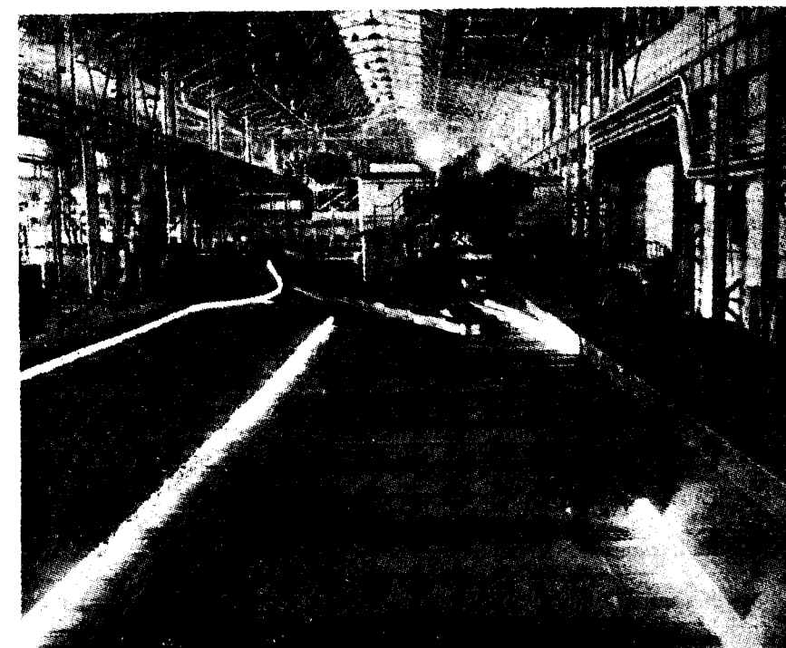
An inside view of the Structural Mill of the Bhilai Steel Plant
