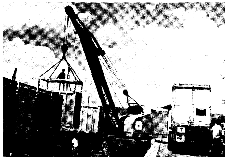
Container-Service in operation
