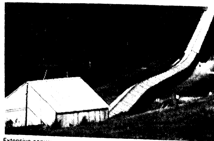
Extensive conveyor system with Siemens drives and controls.
