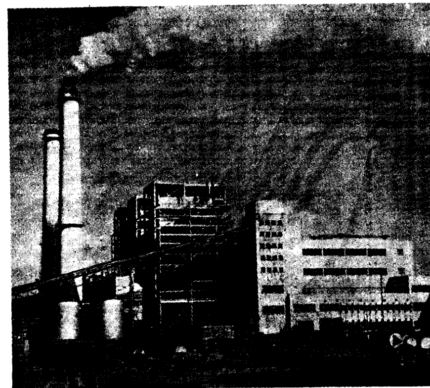
A view of the Chandrapura Thermal Power Station
