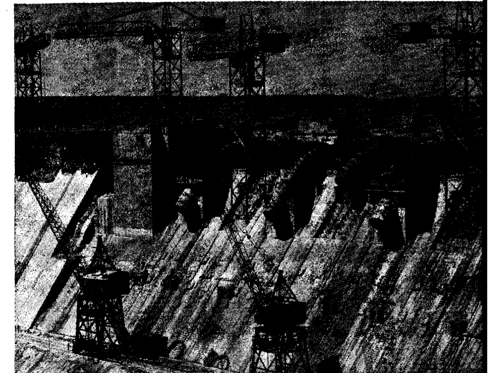
The Nagarjunasagar dam under construction
